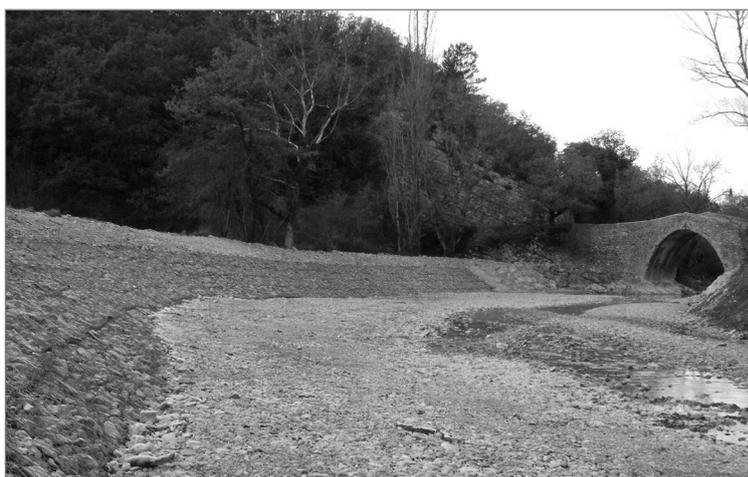
**Figure 3.107** *Gabion protection to a river channel – the bank is exposed to current attack only under high flows during flood conditions*
