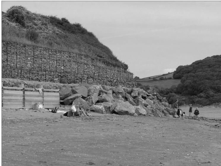
**Figure 3.108** Gabion baskets used as retaining wall behind primary armour
