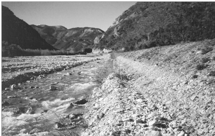
**Figure 3.106** *Gabion riverbank protection*
