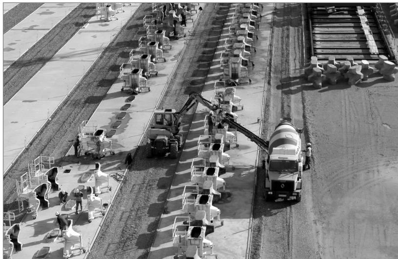
**Figure 3.97** Example of concrete armour unit prefabrication site with preparation of moulds (front left); pouring and vibrating (front right); curing and stripping (back view) (courtesy Port du Havre)
